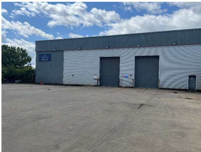
Secure dedicated service yard
